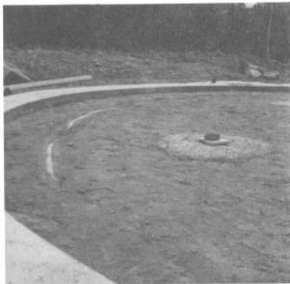
Illus. 5-6. The bottom half of the pillar footings are poured and the concrete is left rough to make a good "cold joint."
