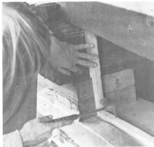
Illus. 12-3. Installing the trapezoidal window in the north wall. Since it was convenient to work from the outside, I fastened the inside molding first.
