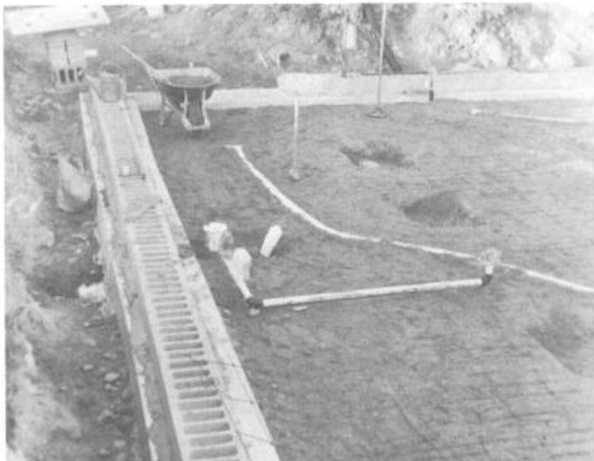
Illus. 5-8. Perforated 4" tubing was laid to remove any water that might accumulate under the floor.
