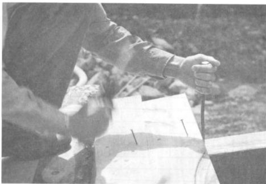
Illustrations 8-2 and 8-3. If you use green wood, nail the planks as shown in these two photos, using a spike to keep them tight against each other, and nailing the lower nails first.
