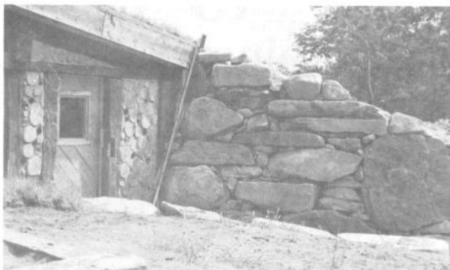
Illus. 13-1. The large triangular spaces left between the boulders can be filled with smaller stones.
