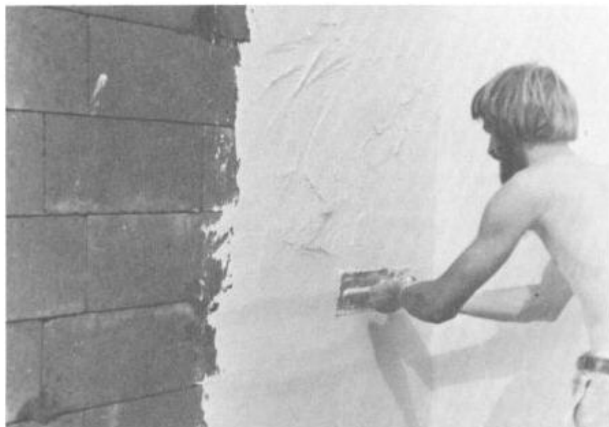
Illus. 6-5. Work the mix onto the wall using a plasterer's trowel.
