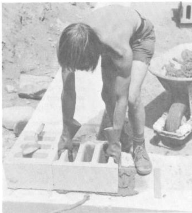
Illus. 5-4. Keep the blocks tight against each other.
