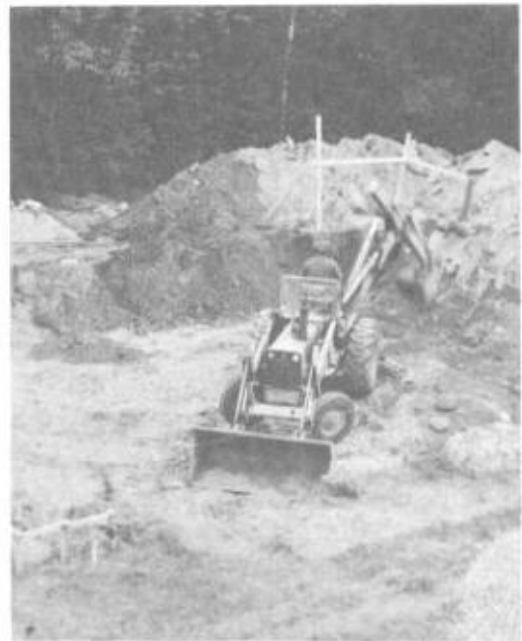
Illustrations 4-1 and 4-2. Excavating a hillside with a front-end loader and its 6'-bucket. The site should be excavated to a flat surface about 2' beyond the outside of the planned footing.
