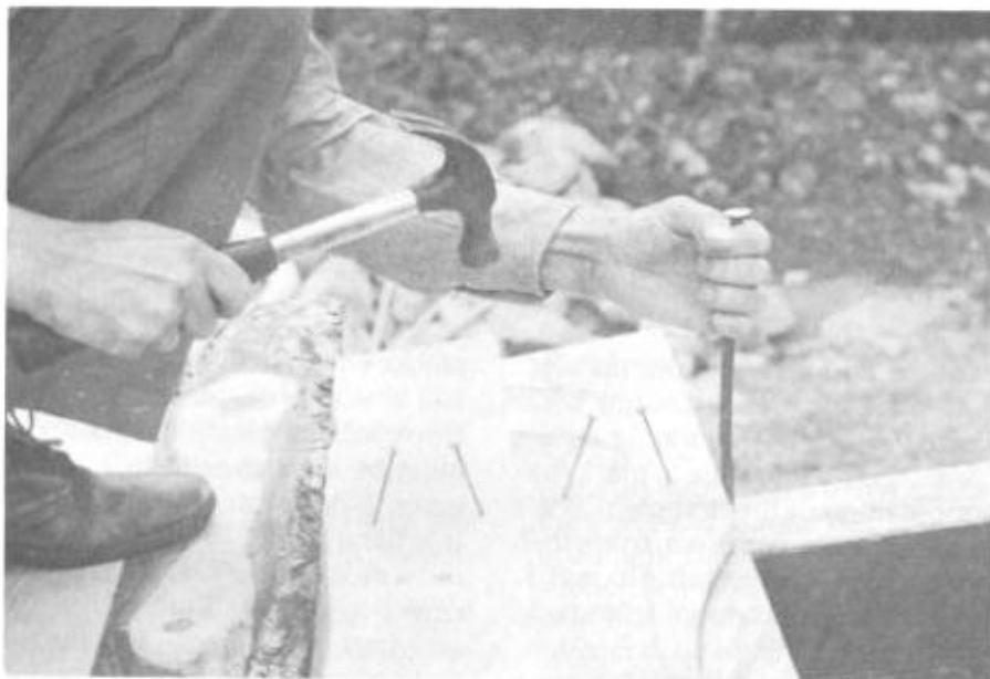
Illustrations 8-2 and 8-3. If you use green wood, nail the planks as shown in these two photos, using a spike to keep them tight against each other, and nailing the lower nails first.
