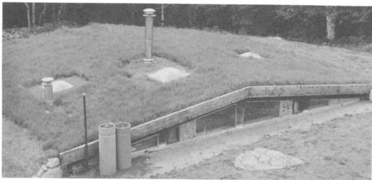
Illus. 13-4. The sod roof is in place. The north gable windows admit light to the back rooms.
