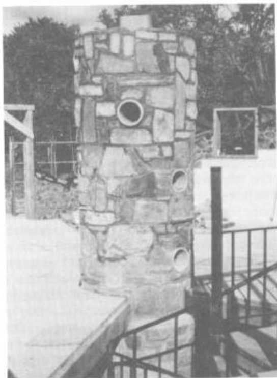
Illus. 14-5. The masonry stove at Earthwood
