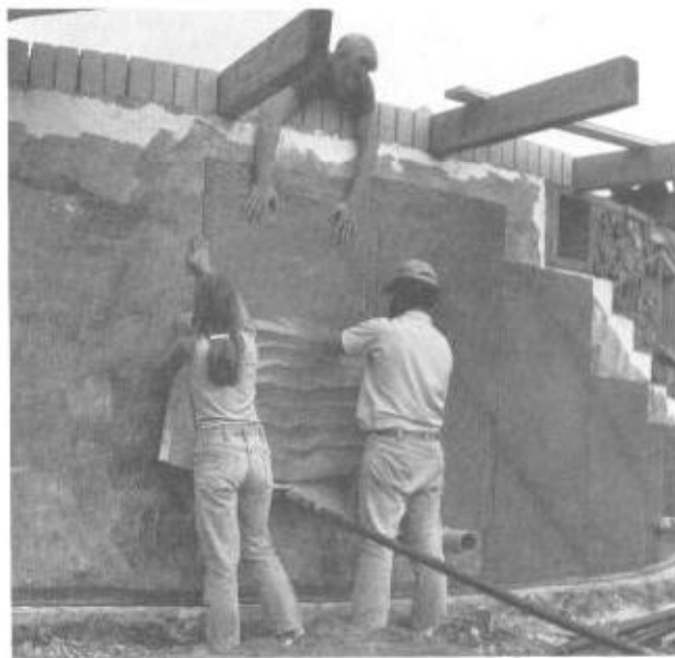
Illus. 9-2. The Bituthene® waterproofing is applied vertically to the walls.
