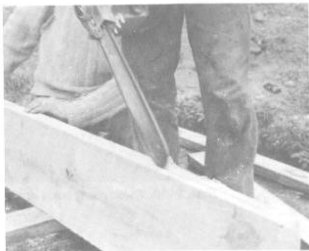
Illus. 8-9. Use a chainsaw to cut a groove down the middle of the fascia board before nailing the board into place. This groove will serve as a "drip edge" to keep rainwater from running along the underside of the roof planking and into the house.
