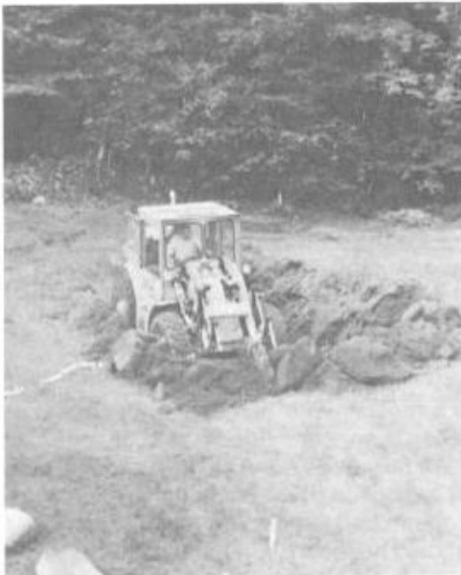
Illustrations 4-1 and 4-2. Excavating a hillside with a front-end loader and its 6'-bucket. The site should be excavated to a flat surface about 2' beyond the outside of the planned footing.
