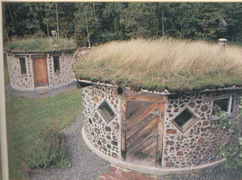
(Left, middle) Earthwood Building School, West Chazy, N.Y. (Left, bottom) Freestanding grass roofs on Earthwood outbuildings
