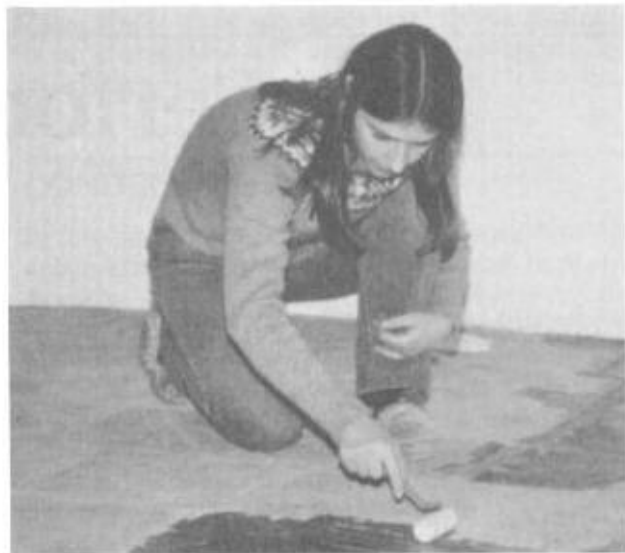
Illus. 14-7. Jaki, at Earthwood, seals the floor, which is made of roofing slates set in strong mortar:
