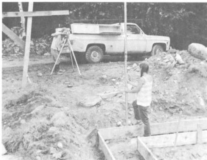
Illus. 4-9. The most important consideration when placing the footing forms is that they be level with one another.
