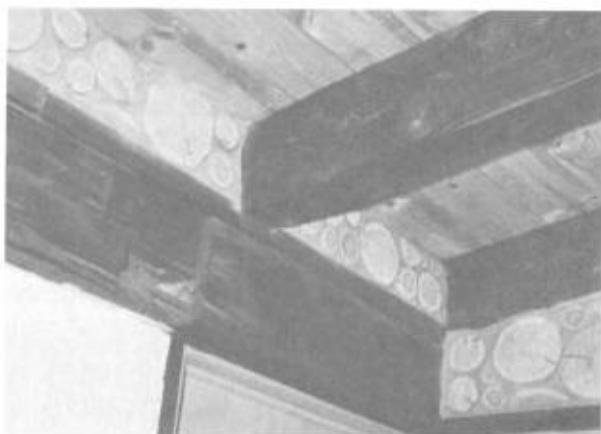
Illus. 14-2. Log ends fill the space between rafters from the top of the beam to the roof planking. They go well with the rough-hewn style of the house.
