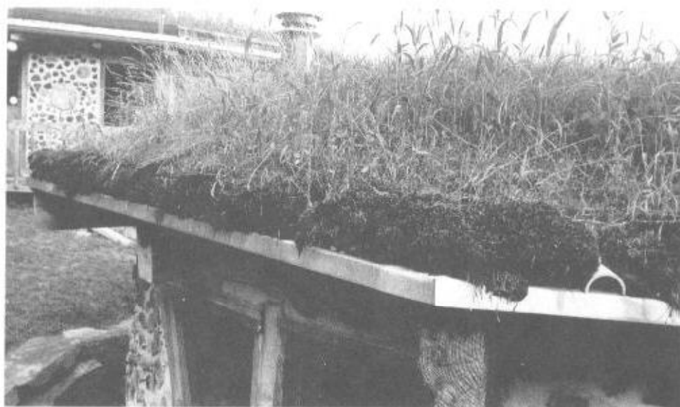
Illus. 8-10. These moss sods drain well, retain the earth, and look natural.
