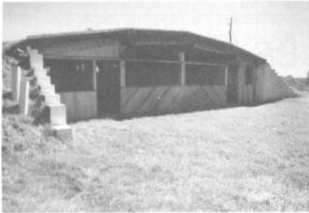
Illus. 17-1. An early look at Becky and Roger's underground house in the "Deep South" (Becky Gillette photo)
